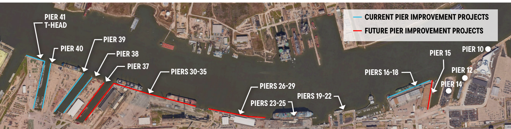
FIGURE 1: GALVESTON MASTER FACILITY ASSESSMENT
